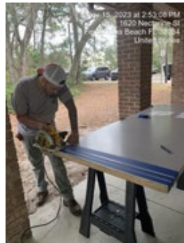
Trimming door to be hung at the Health Department
