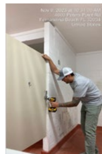
Repairing a latch on the men's restroom stall at Peters Point Beachfront Park
