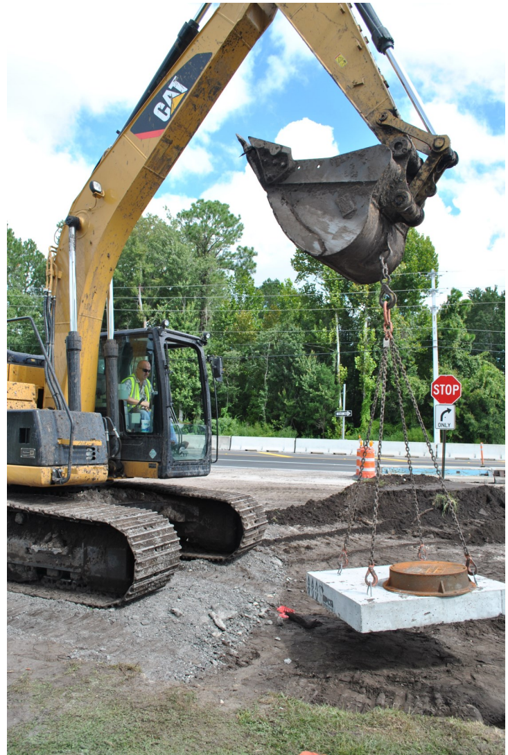
Drainage structure installation underway on A1A
