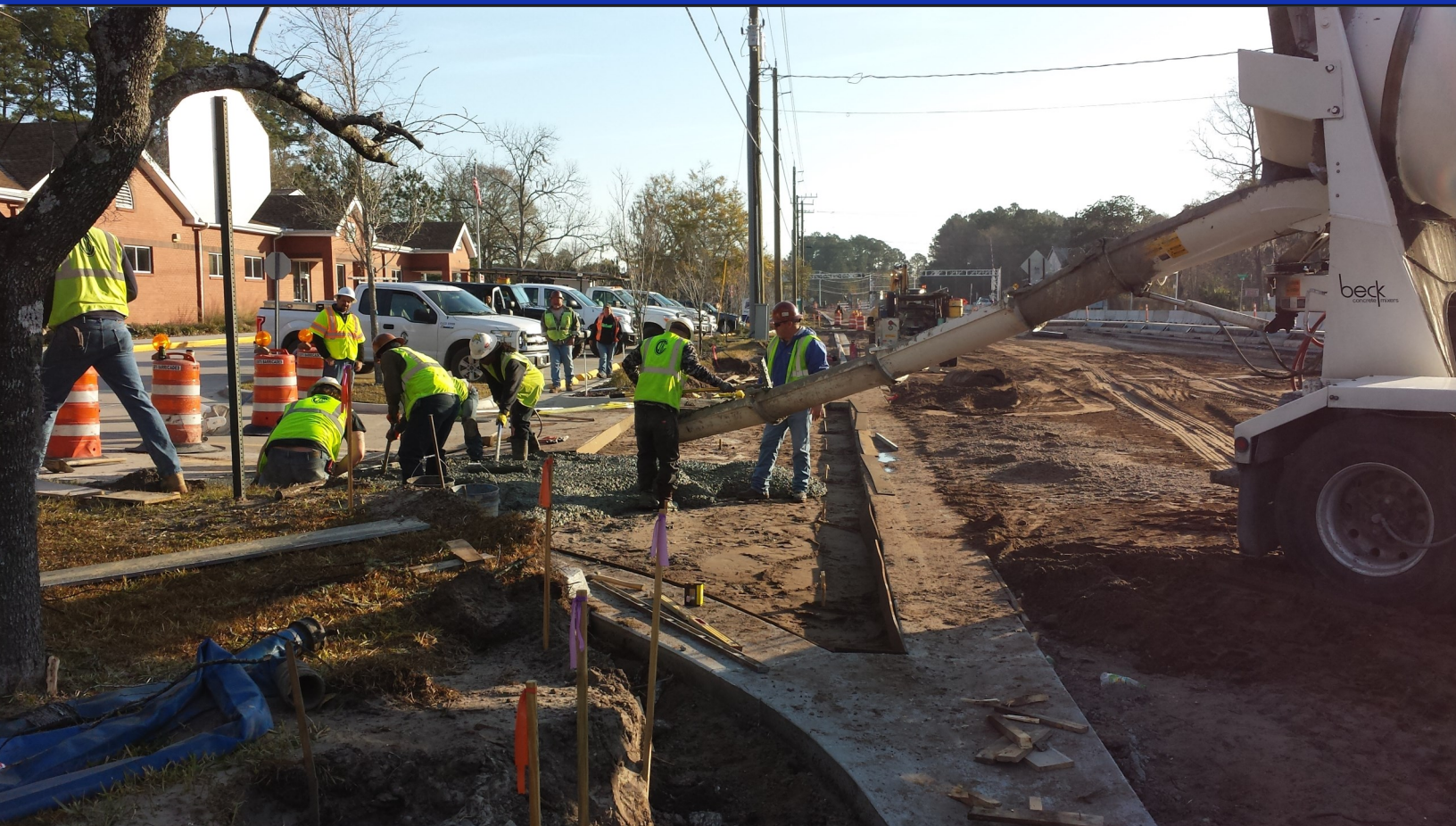
Workers from J.B. Coxwell pour concrete on A1A project in Yulee.
