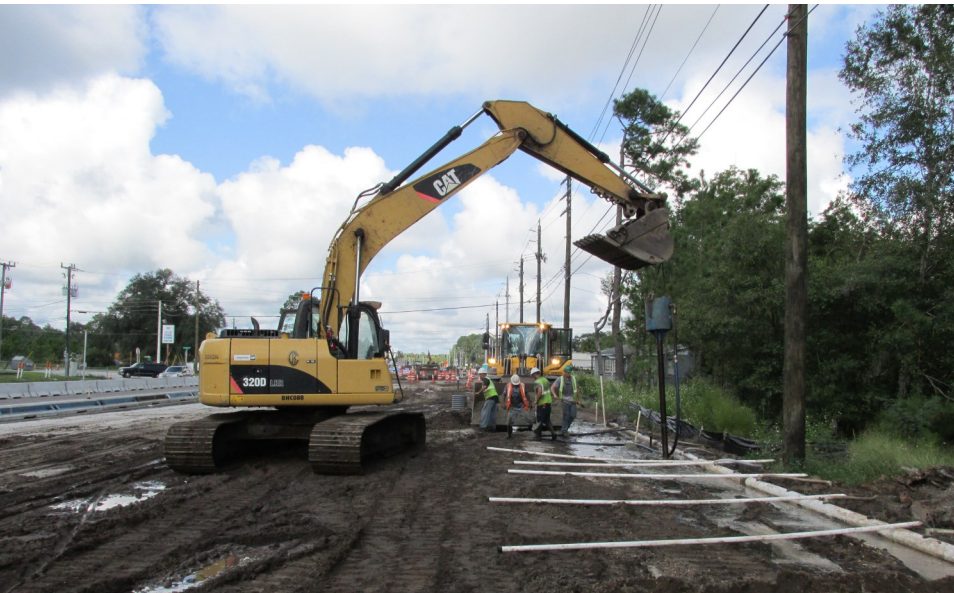
Temporary pipes are placed along the road to help with drying the area for excavation.
