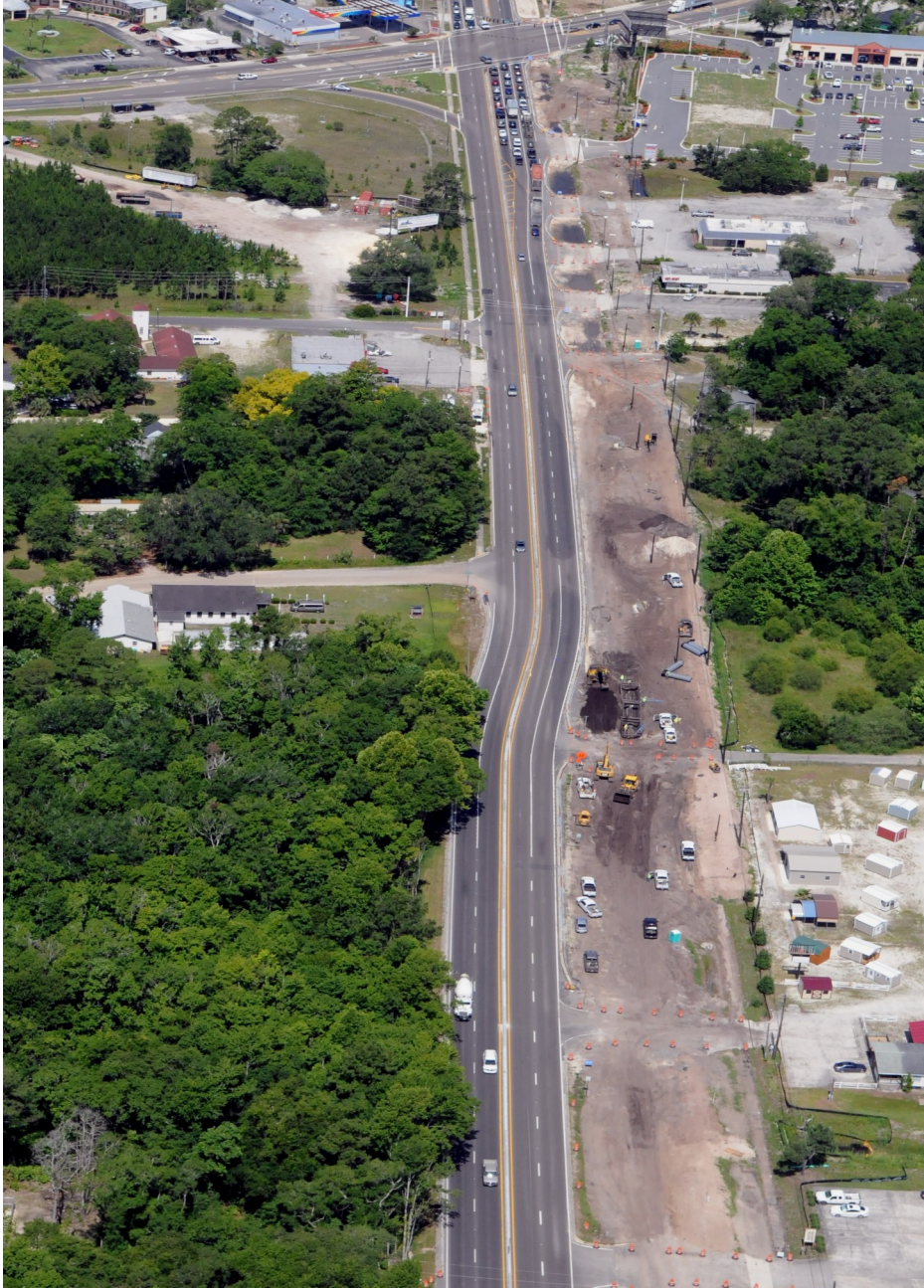
Aerial view of the construction work area for the widening of State Road A1A.
