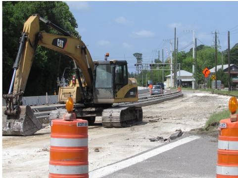
Old asphalt is removed from the westbound lanes along with road base construction near the post office.
